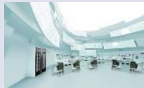
Distributed control systems
